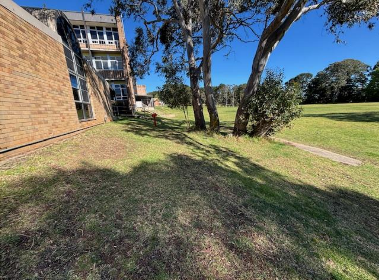
Photo A: Additional information is required in terms of existing and proposed levels around trees 14, 15 and 16 to determine the development impact.
